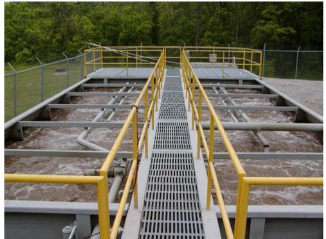
Figure 4) Center Catwalk and Hand Rail (optional Clarifier Perimeter Hand Rail)
