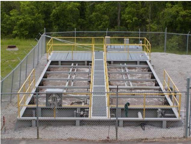
Figure 3) 60,000 gpd WWTP with Sludge Digester
