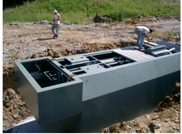
Figure 2) Full galvanized service grating being set
