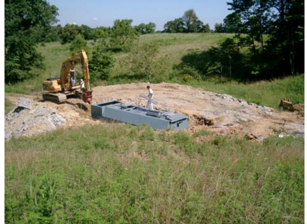
Figure 4) Backfill operation beginning
