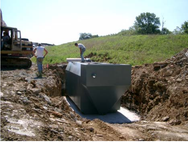
Figure 1) Just after WWTP was set
