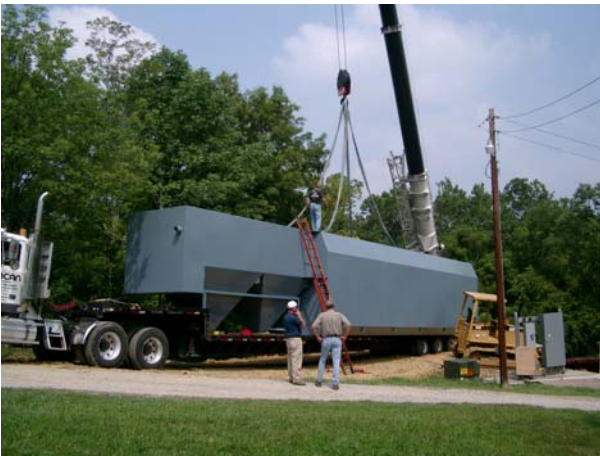
Figure 3) Rigging the WWTP for the lift
