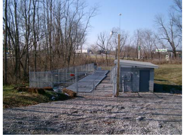
Figure 2) WWTP Site showing Concrete Block Building
