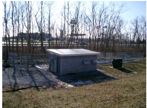
Figure 4) Concrete Block Building showing rain shields over blower intake filters
