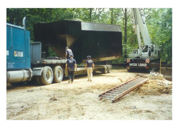
Boy Scouts of America, Camp Friedlander 8,500 gpd Package Plant to include Flow Equalization and S.H.T. Site Built Slow Sand Filter and Sludge Drying Bed (Not Shown)
