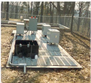
Boy Scouts of America, Camp Friedlander 8,500 gpd Package Plant to include Flow Equalization and S.H.T. Site Built Slow Sand Filter and Sludge Drying Bed (Not Shown)
