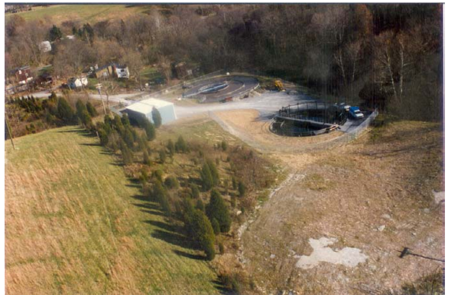
Alexandria Treatment Plant, Campbell Co., Ky. Sanitation District #1, Ft. Mitchell, Ky. 1 st Stage – Partial Ring Addition 2 nd Stage – Circular Clarifier, S.H.T., Chlorination
